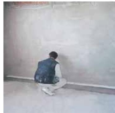
The first layer, the **rendering coat**, has a thickness of 15 -20mm using coarse sand; it is applied in place with a trowel, creating a homogeneous and rough surface. The **puckering coat** is made to a thickness of 10 - 12mm using medium-grain sand, waiting until the first coat is sufficiently dry.
